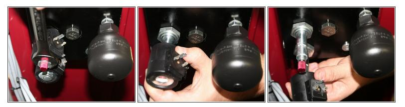
• Remove both 24VDC coils from solenoids on back of old control manifold.
